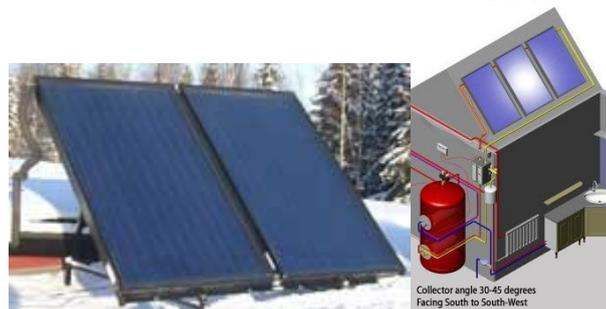
Fig. 3.7: Sun collector system provided by Rica can be used for water heating [Rica, 2012].
