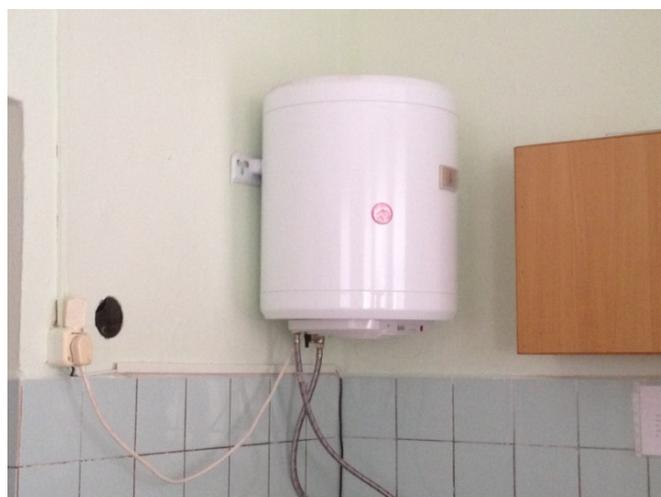
Fig. 7.3: One of the electric boilers used to heat domestic water.
