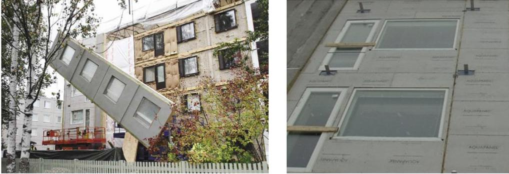
Fig. 3.1: Paroc's passive house concept is based on prefabricated facade elements with substantial insulation and energy efficient windows [Paroc, 2012b].
